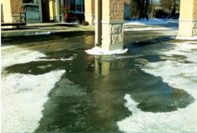
The Smart About Salt program encourages property managers to identify problem areas that will require excessive amounts of de-icing salt, and correct them. Here, improperly installed roof drains flow over a pedestrian area and parking lot where the water can refreeze, causing icy conditions.
